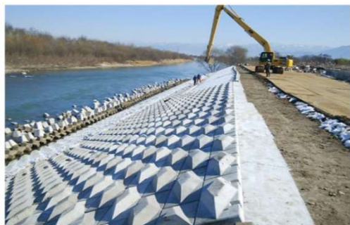
若穂牛島・四ツ屋護岸災害復旧
